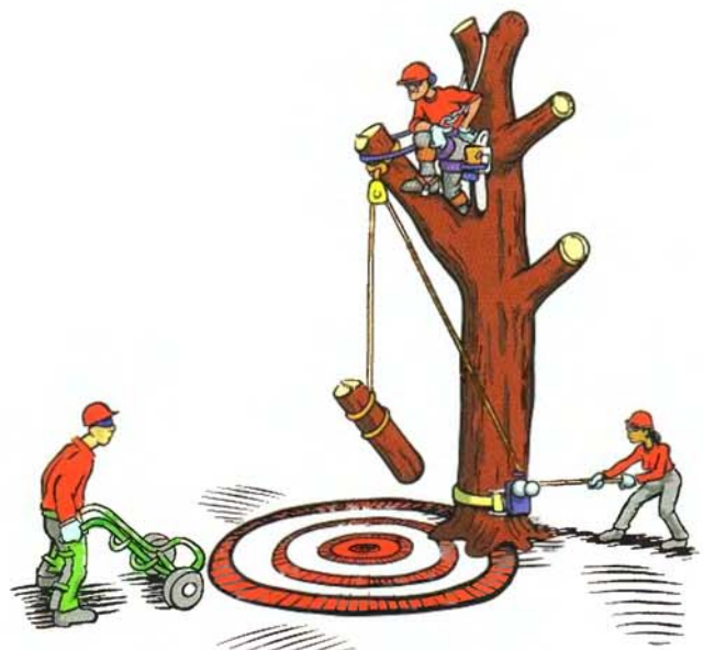
FIGURE 2.9 Workers must know when it is safe to enter a work zone. The voice command-and-response system is a good way to maintain safety.
